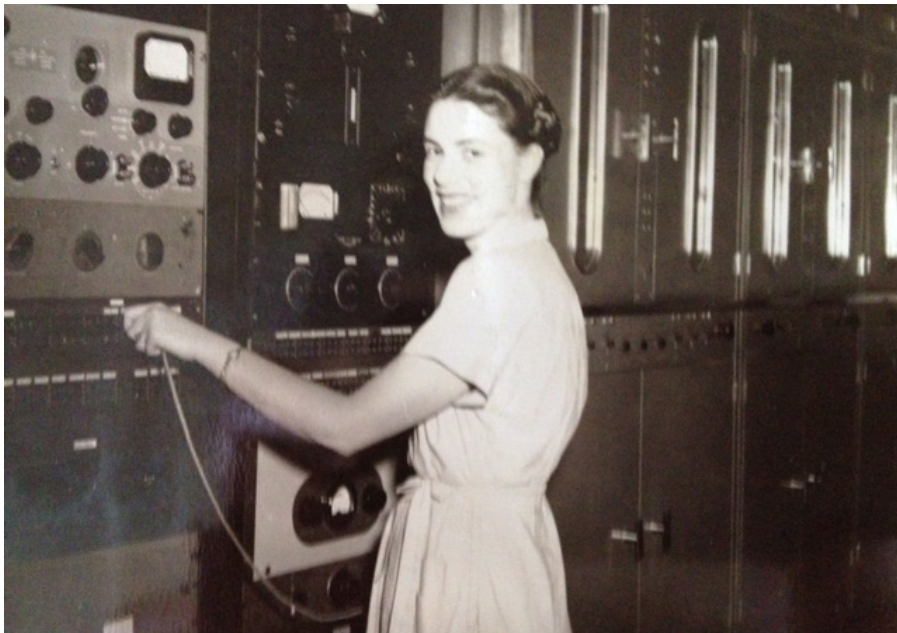
Ellen as KPOA station engineer.
